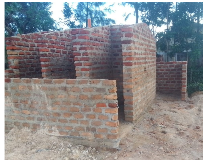
The progression of latrine construction from digging the pits, lining the pits with brick, and then the above ground construction
