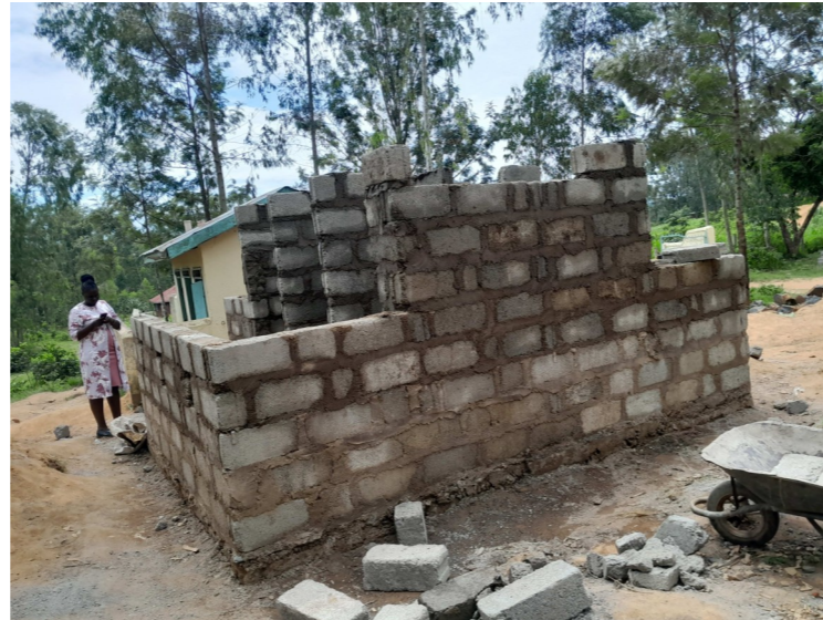
The progression of latrine construction from digging the pits, lining the pits with brick, and then the above ground construction
