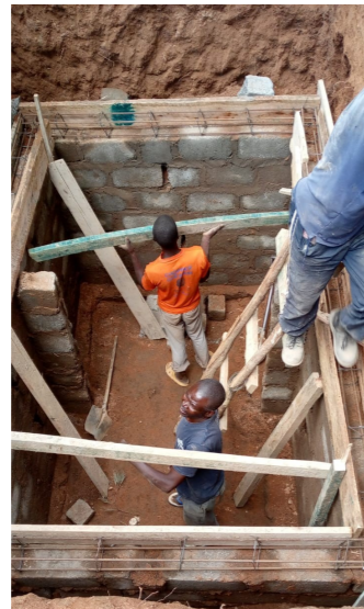
The progression of latrine construction from digging the pits, lining the pits with brick, and then the above ground construction
