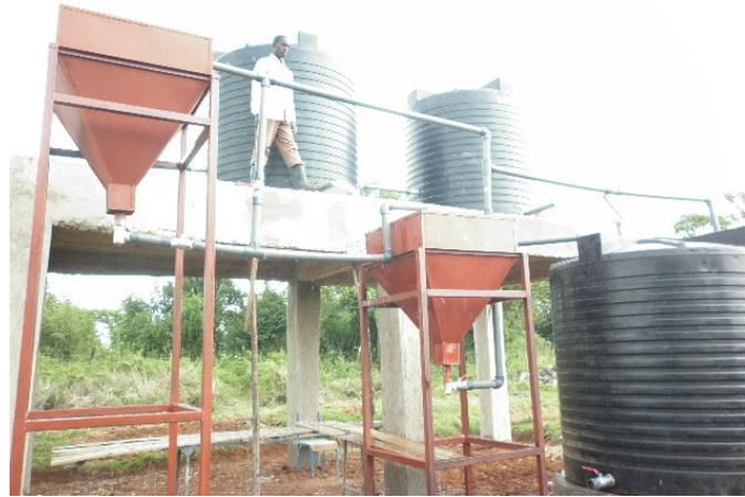
**Stage three of the project. Water Purification via a two-stage Filtering process**
