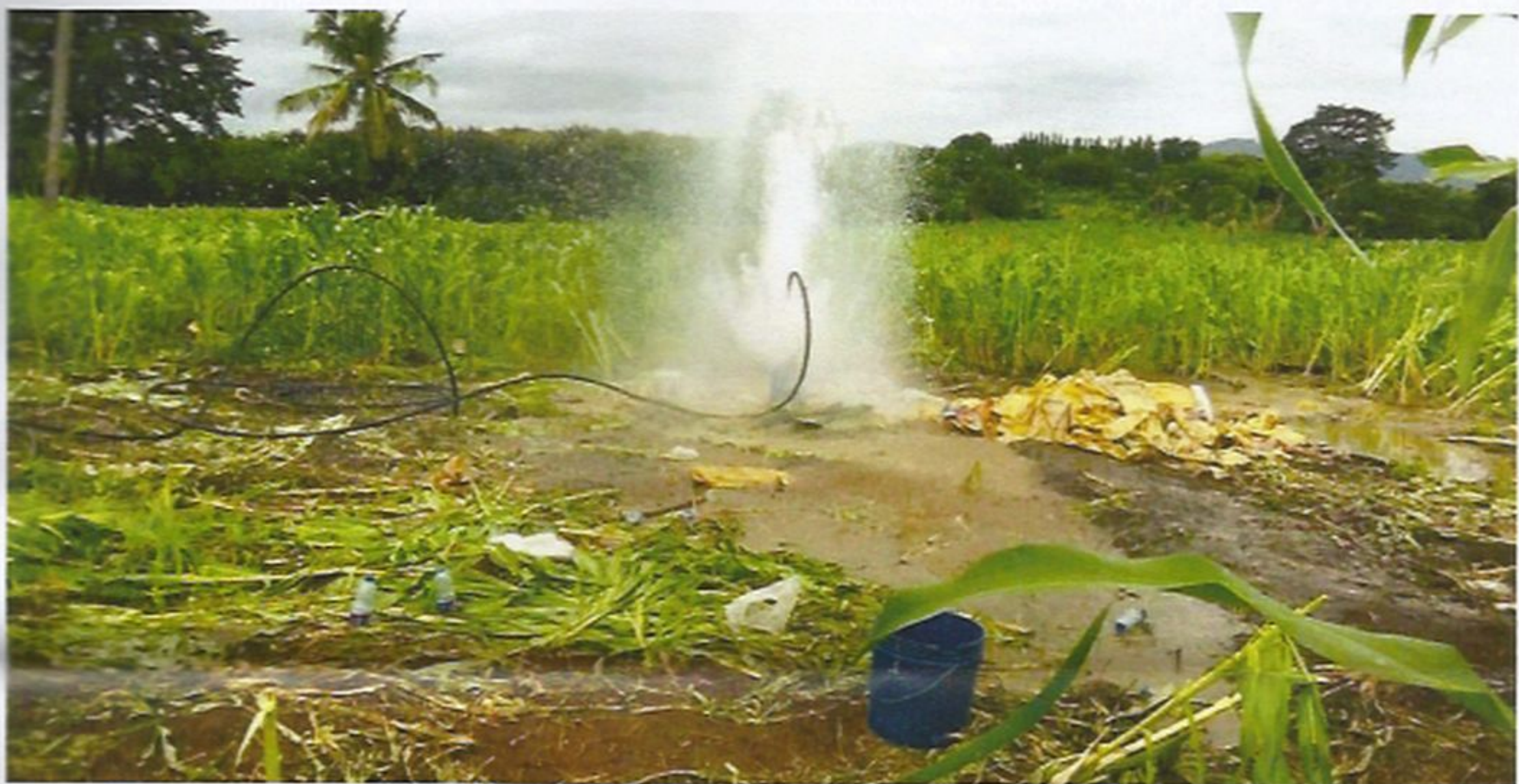
Hitting the prize! Water comes gushing as the well is reached.
