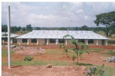
Three-classroom Form IV block built in Tanzania in 2011
